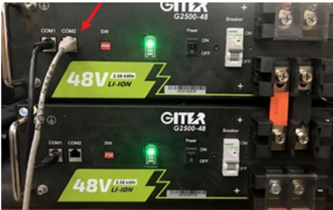
Figure 1: COM2 port for Giter Battery
